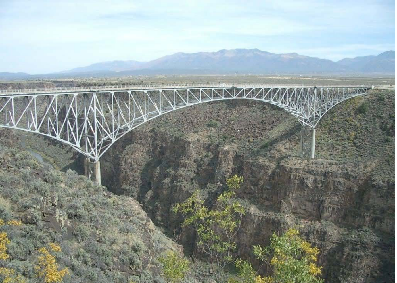
The Rio Grande Gorge Bridge is a cantilever truss bridge over the Rio Grande, in New Mexico, 650 feet below. It was completed in 1965 and was once named Most Beautiful Steel Bridge in the Long Span category by the American Institute of Steel Construction.
