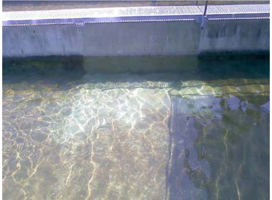
SDS-BIONIC Marine & Hull Coat after 2 months
